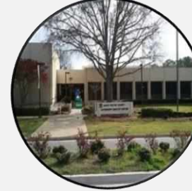
General Services Facilities
